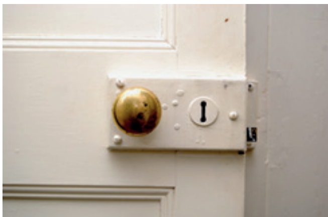
A typical Victorian panelled door in a house: upgrading to provide half-hour fire protection could be achieved by the use of intumescent perimeter seals and intumescent paper to the recesses of the panels with minimal impact on its character.
